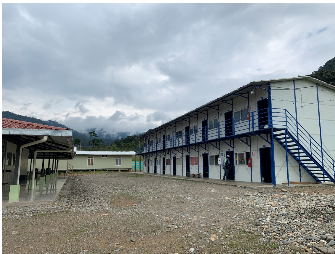
Figure 1 – Camp facilities acquired for El Domo construction, including accommodations for 100 personnel
